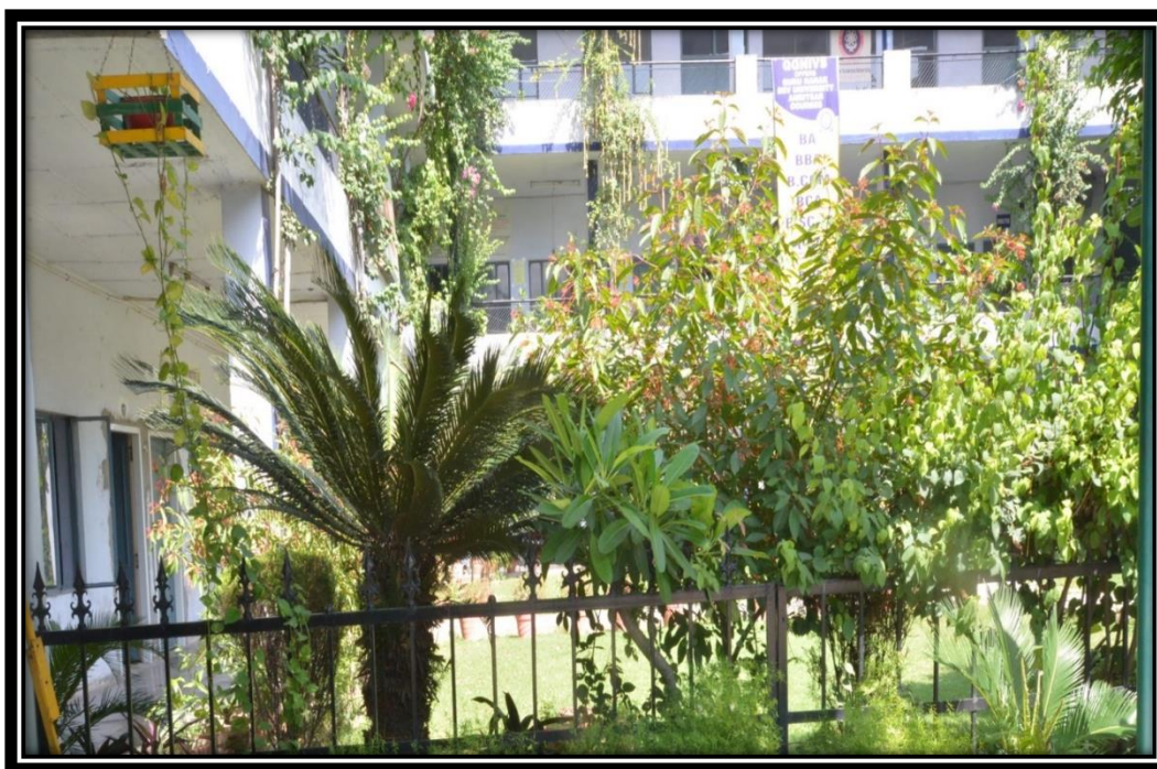
Climbers Growing in the Lawn Adjacent to Administrative Block.
