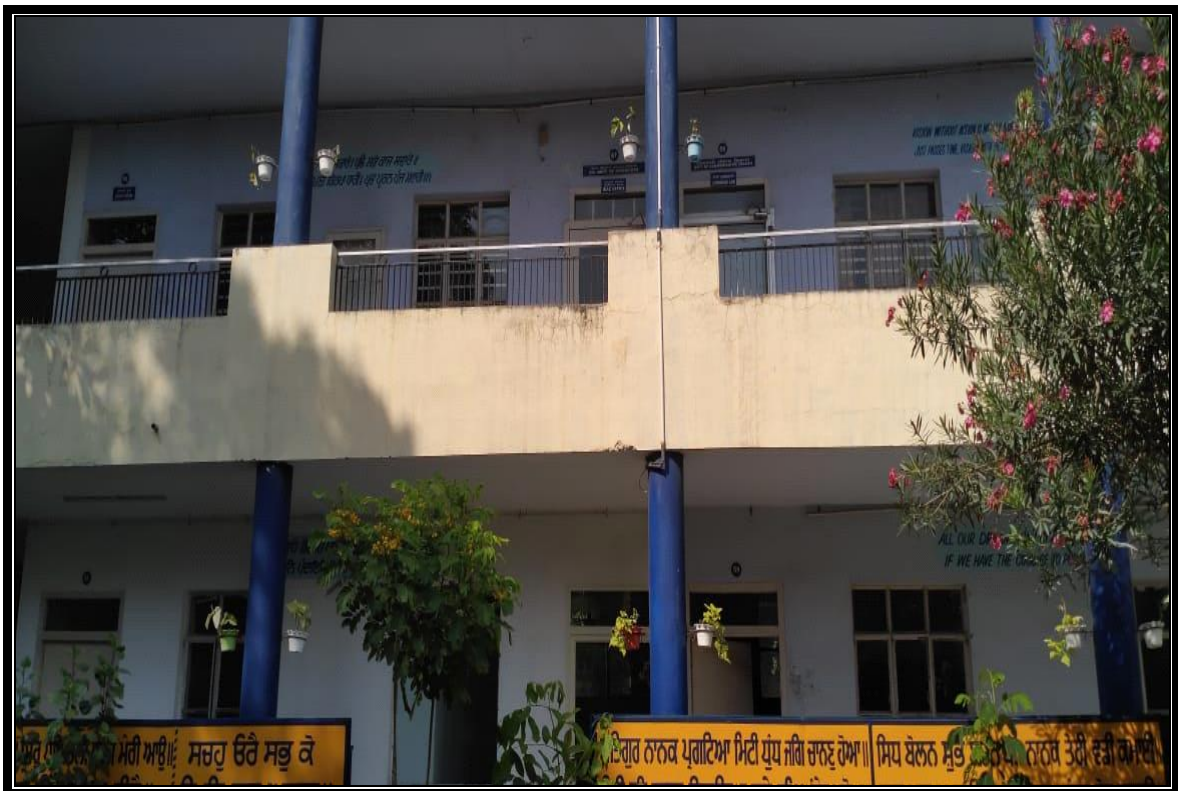
Flower Pots Installed on Pillars in Golden Jubilee Block.
